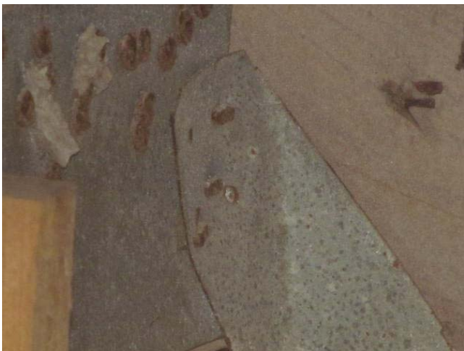
Clips - with minimum three nails
